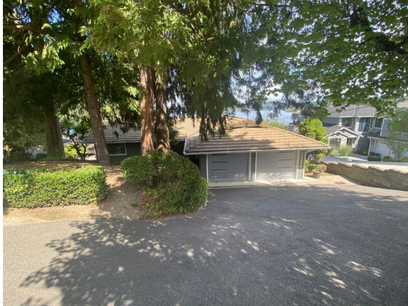
Plate 1. View of the west side of the existing residence and garage at the site, looking east from North Mercer Way.
